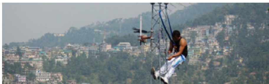
Figure 11.5: Dharamsala installer working on a tower
