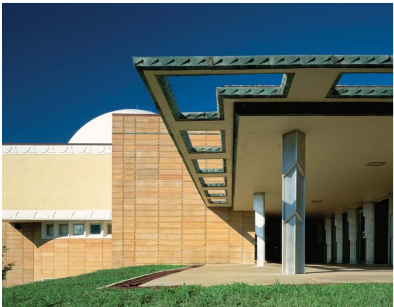
Original solar shading by Frank Lloyd Wright
