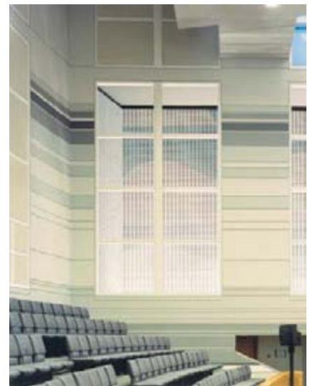
Acoustical 'cloud' wall. (See also the third plan above)
