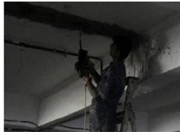
**Figure 5.** Epoxy injection in progress
