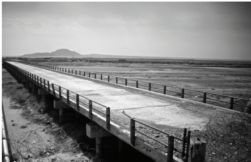
Arghestan Bridge, Kandahar province
